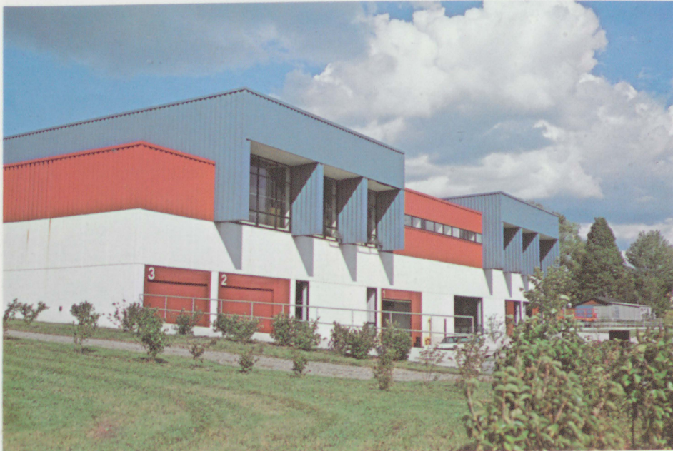
Brewer's modern waste water treatment plant
