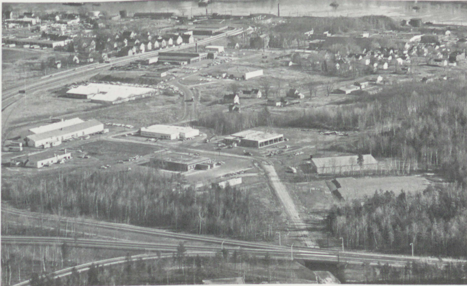
Many of the area's industrial parks are near Interstate 95.
