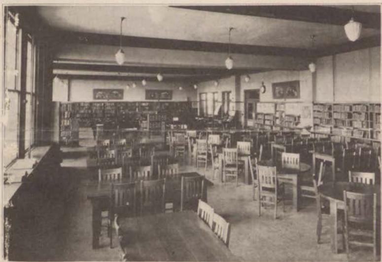
North Central High School Library, Spokane, Washington View from main desk
