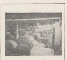
Above photo taken in the beater room of the Eastern Mill showing the way in which the pulp is mixed. When colored papers are made the dye is put into these tanks with the pulp and thoroughly mixed.
