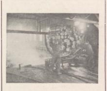
Photo showing handling of wood from tracks into soaking tank. This method is not in use at the present time but was used for steaming the wood especially in winter to remove the frost and ice. Our more modern method for doing this is a large concrete tank into which the wood is dumped directly from the pile and saves handling on a track.
