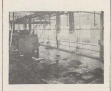
This photo taken within the mill shows method of bleaching pulp. The receptacles shown at the sides of the picture are tile lined vats into which the unbleached pulp is put to be bleached.
