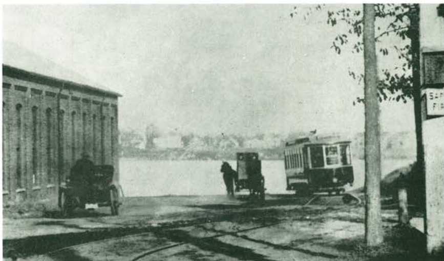
SHOO-FLY track carried the South Portland cars around the rear of the Knightville car barn while the new South Portland bridge was being constructed in 1915-16. —Photo from C. D. Heseltine.
