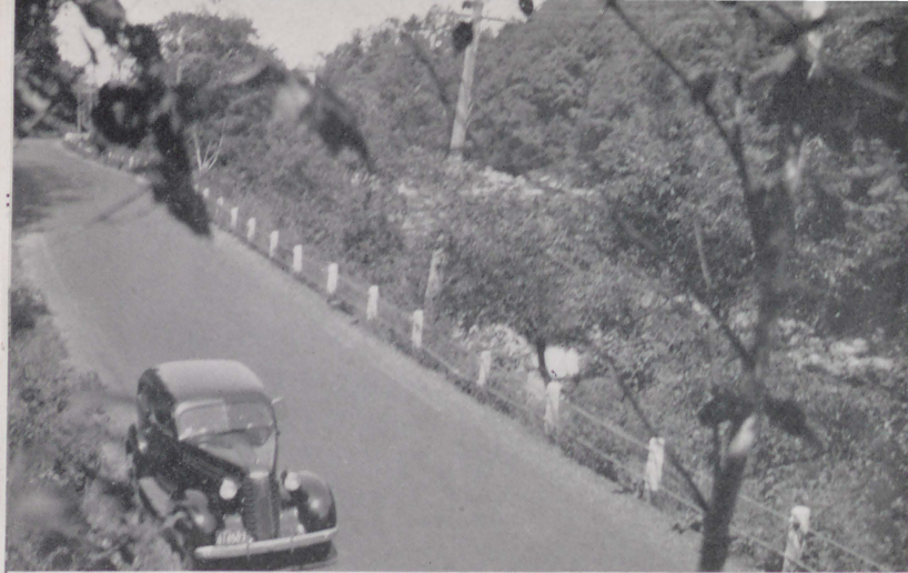
Valley Avenue near Lovers' Leap. Retaining Wall rebuilt
