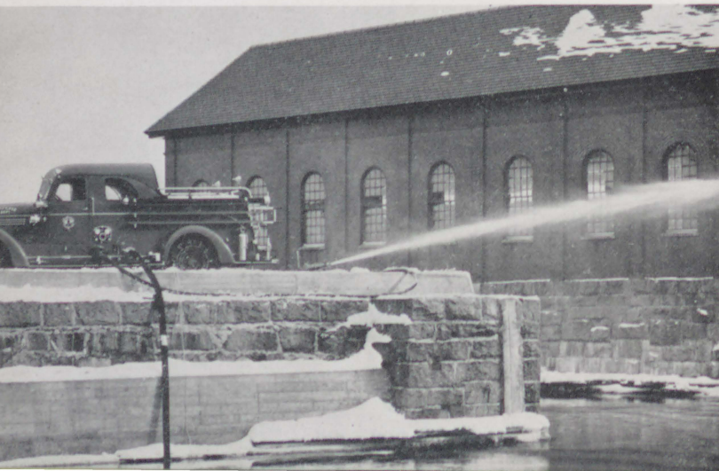
Bangor Fire Department's latest undergoing Fire underwriters' test
