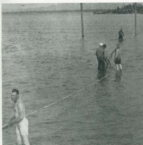
Laying submarine cable
