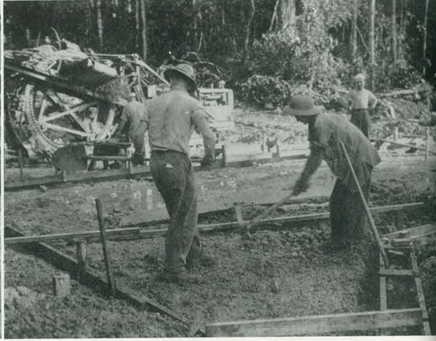
Laying the Chow Hall Foundation at Hollandia
