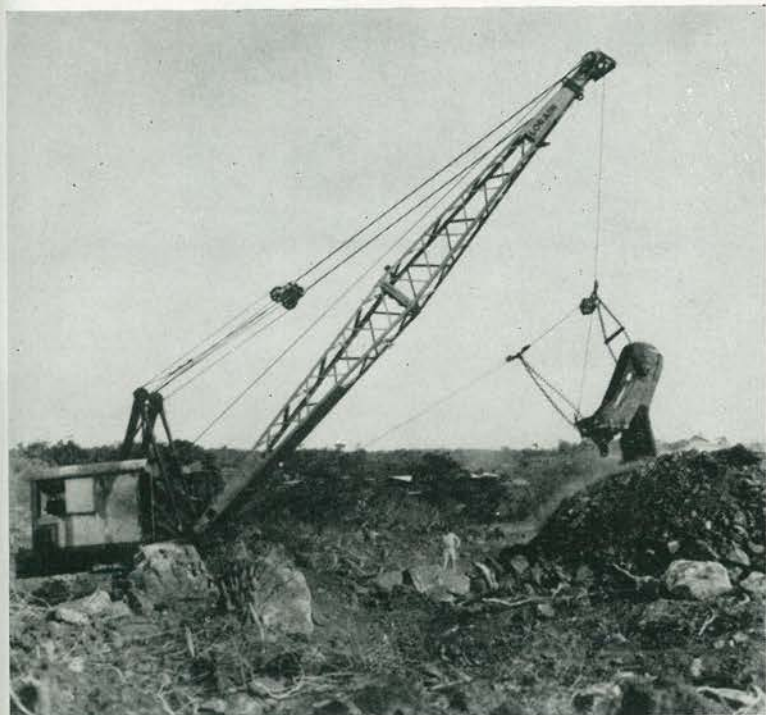
Ditching with Drag Line
