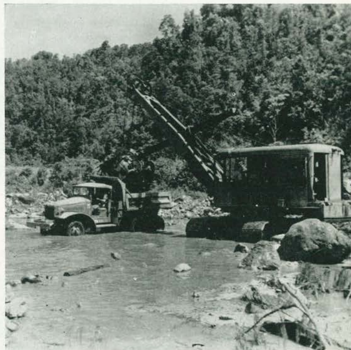
Loading gravel from river bed
